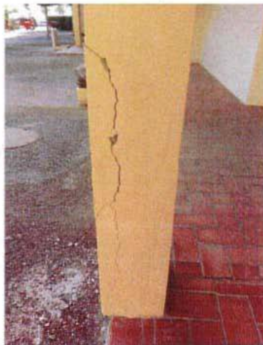
Fissuration piliers
