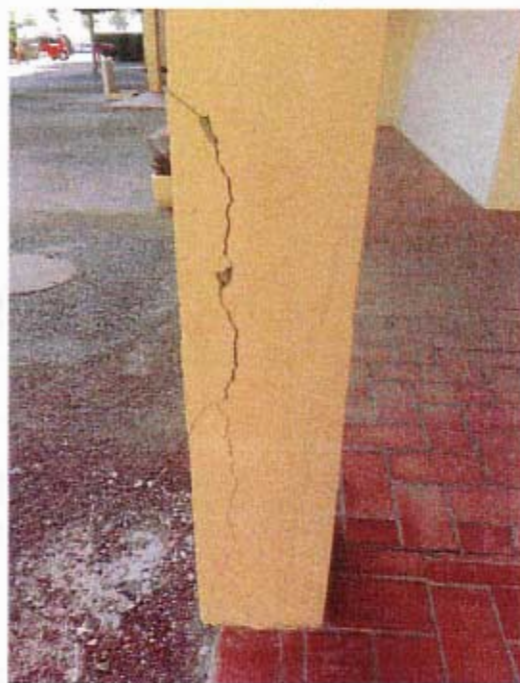
Fissuration piliers
